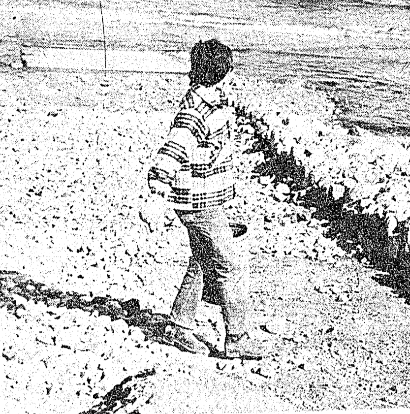
TOTING A BUCKET OF BEACH STONES to ballast a boat launching ramp under construction on Island View beach, this anonymous gentleman is working on a Local Initiatives Programme organized by Mr. Lanny Yee. The stone fill base will be coated with concrete to protect it against erosion. (Review Photo by Gordon Ewan)
