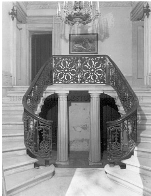
Figure 39: Aiken-Rhett house 1830's addition of entry staircase that reaches from first to second floor, HABS
