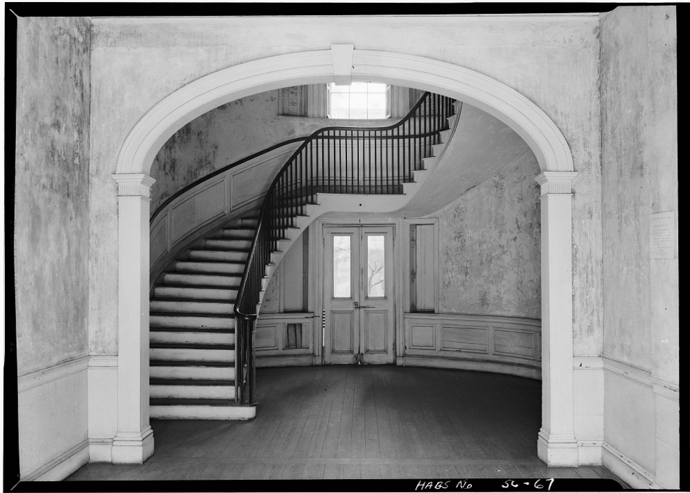
Figure 28: Joseph Manigault cantilevered staircase, HABS
