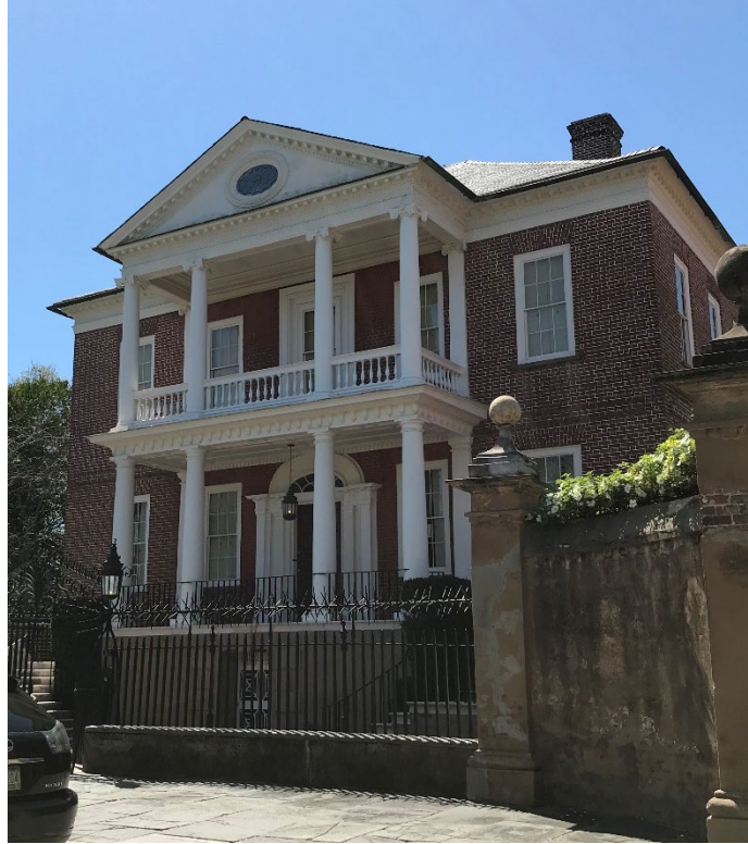
Figure 18: Front façade of the Miles Brewton house, photo by the author
