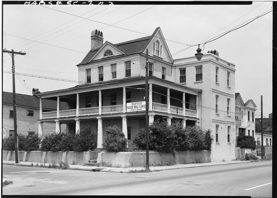
Figure 31: Christopher Belser dwelling southern façade, HABS
