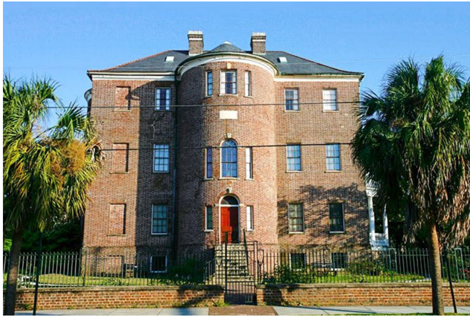
Figure 29: Joseph Manigault house front façade, South Carolina Picture Project
