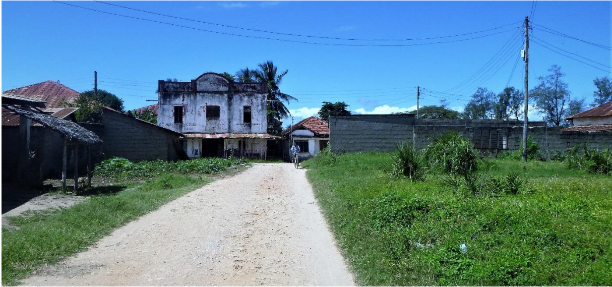
Street view in Pangani with one of the town's old Omani buildings.
