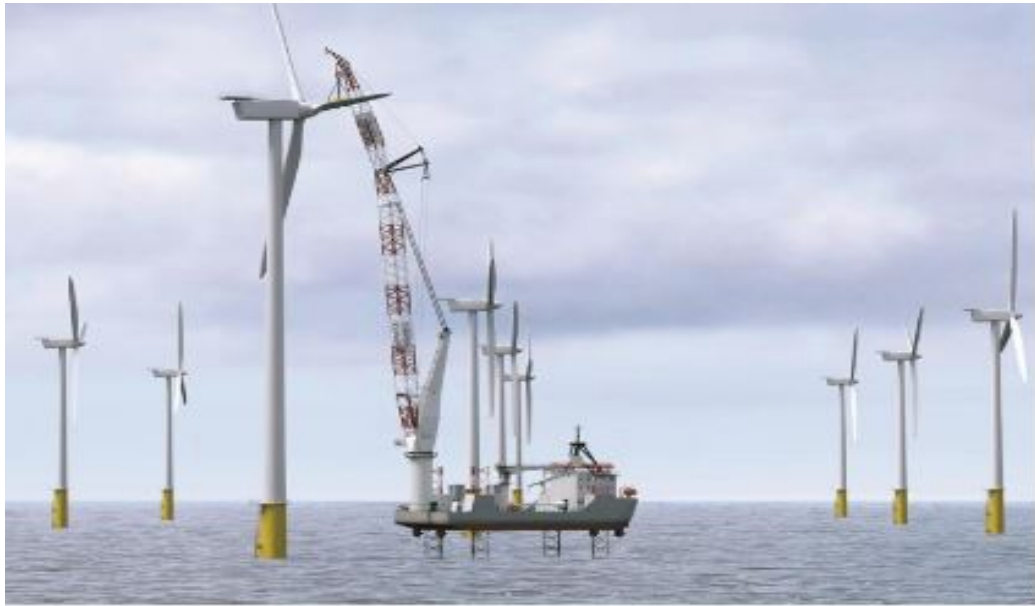
Figure 2.6: Offshore crane vessel for heavy lift[19].
