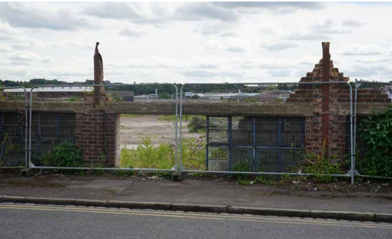
Fig. 14. Former Royal Doulton site, Burslem where plans to develop 140 houses have been put on hold since 2012
