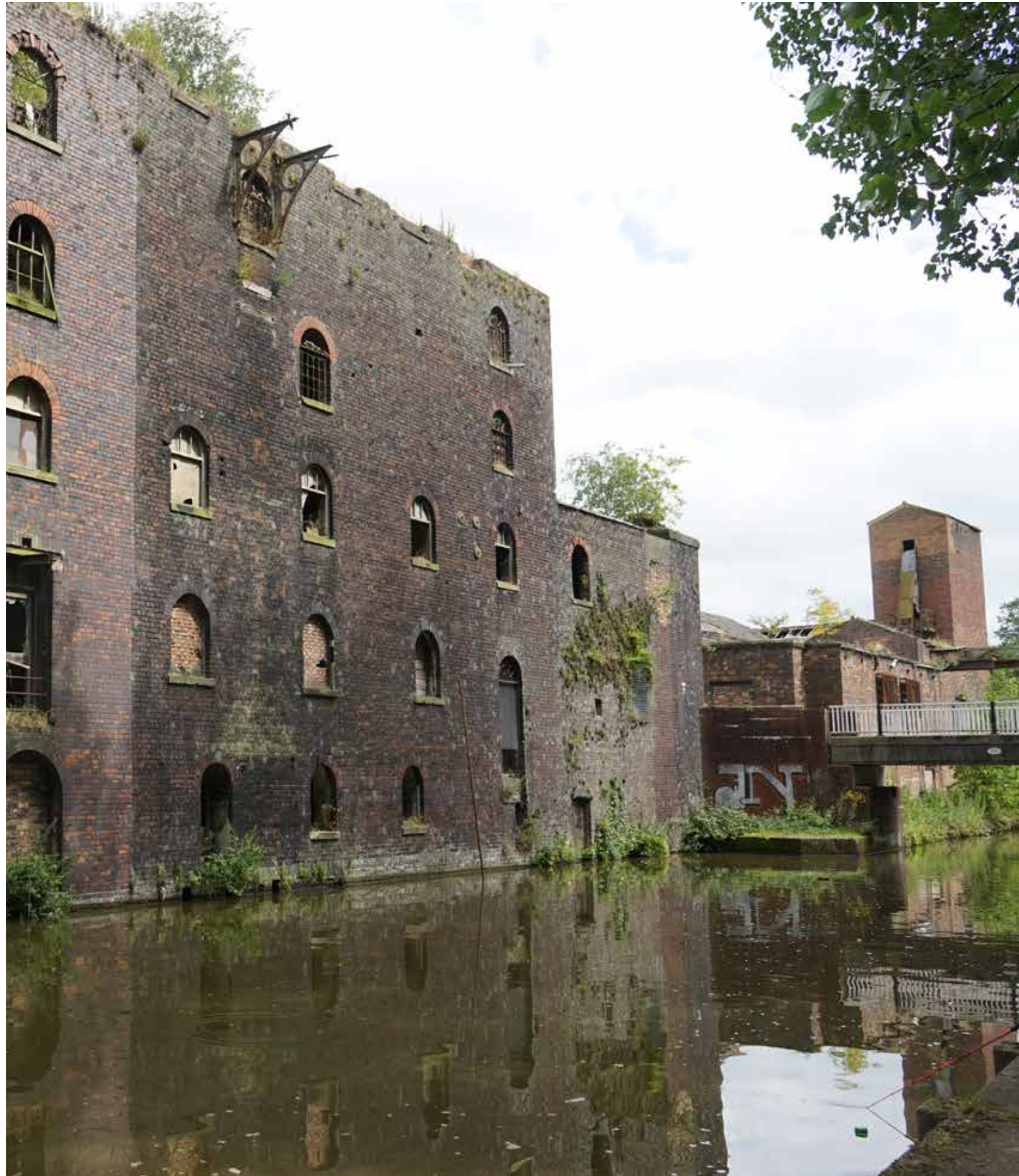
Fig. 1. Former mill and calcining works, Middleport, Stoke-on-Trent, 2015
