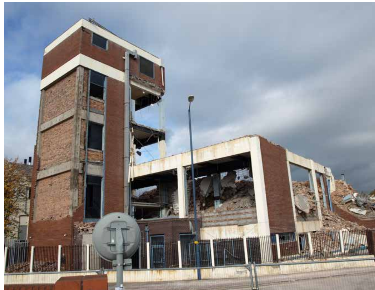
Fig. 4. Former Royal Doulton Nile Street Factory, Stoke-on-Trent in the process of demolition 2008
