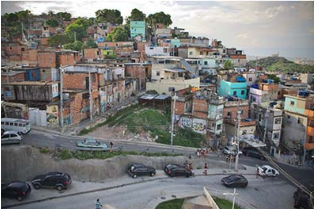
Figure 1: Street life in Complexo do Alemão, a group of favelas in the North Zone of Rio de Janeiro (© Tomas Salem)
