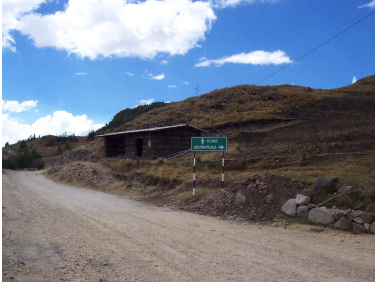
5.7 Road between Tual and Cince.
