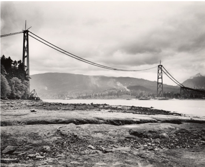
LF.02722, Lion's Gate Bridge mid-construction, undated.
