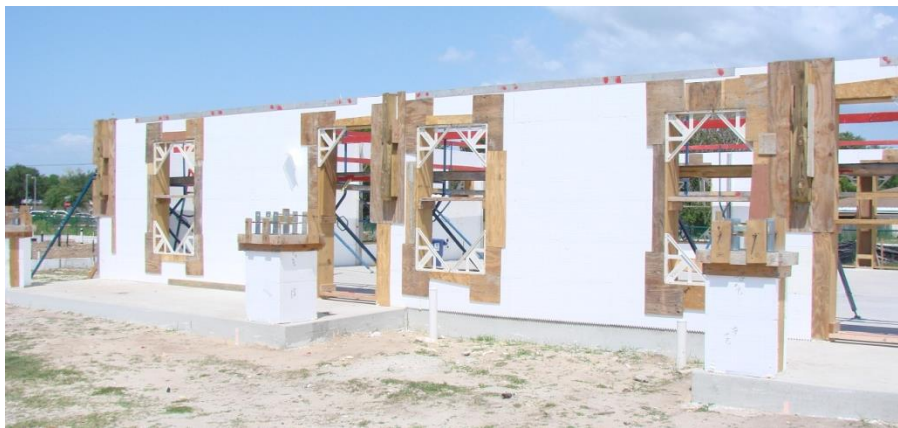
Figure 3. MCHFH ICF exterior wall under construction.
