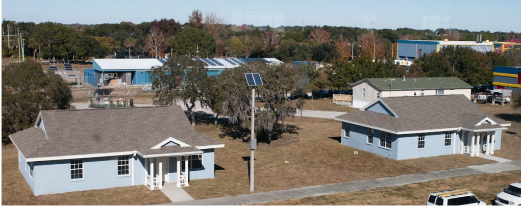
Figure 1. Completed flexible residential test structures on FSEC campus
