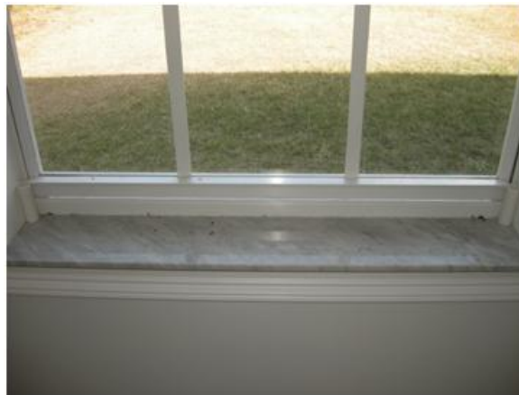
Figure 3. Metal stand-off shims used to add vertical plane leakage to the east building
