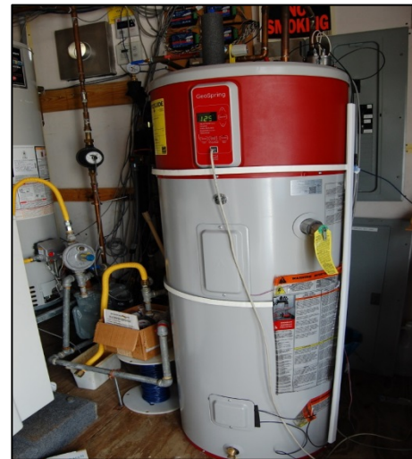
Figure 3.6: Foam rings applied prior to tank shell insulation layer
