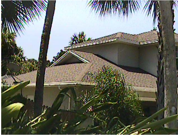
Figure 134 East and north side of house with attic over garage adjacent to open floor cavities.
