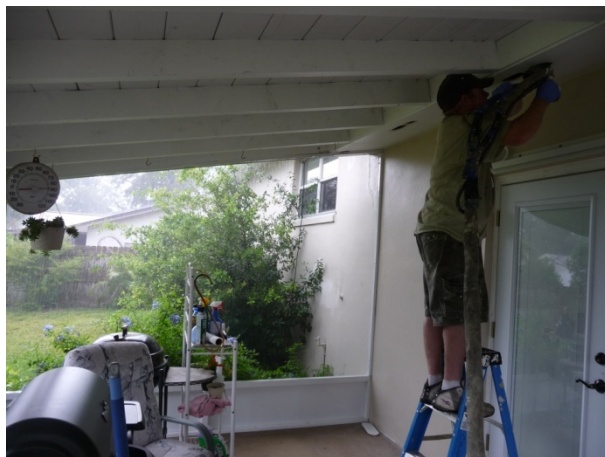
Figure 125 Insulation tech applying insulation through soffit vent openings.
