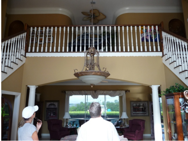
Figure 95 Foyer grand staircase had more cracking on the right side stairs which is closer to most of wind washing areas.
