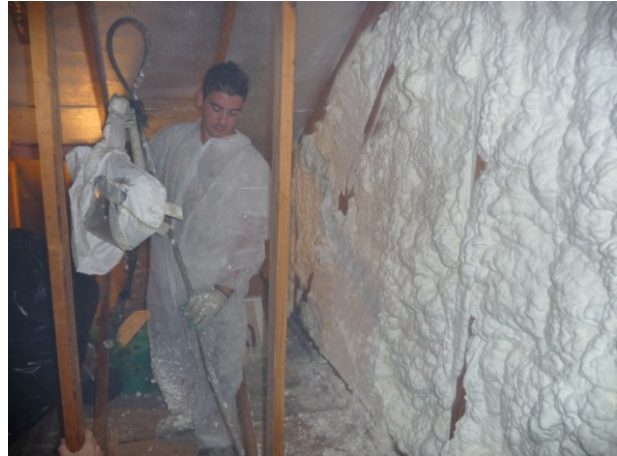
Figure 111 Insulation tech just finishing up kneewall and floor insulation/ air tightening.
