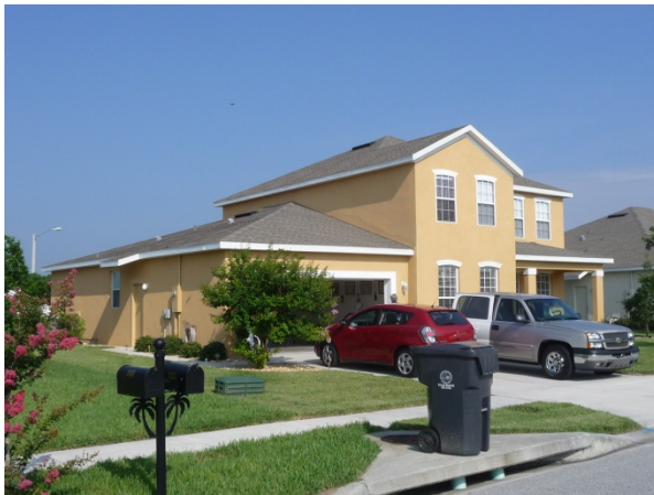
Figure 157 H19 Exterior view of home.
