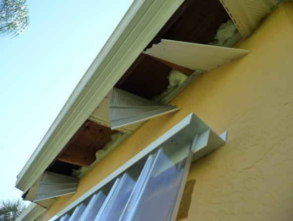
Figure 102 North soffit area after foam installation.
