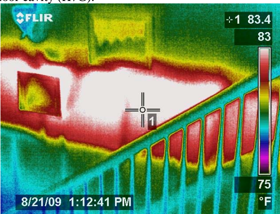
Figure E-9 Infrared image of floor space behind wall in house H23. Wall surface is about 83.4F at floor space due to open floor space to attic on east and west sides of house.
