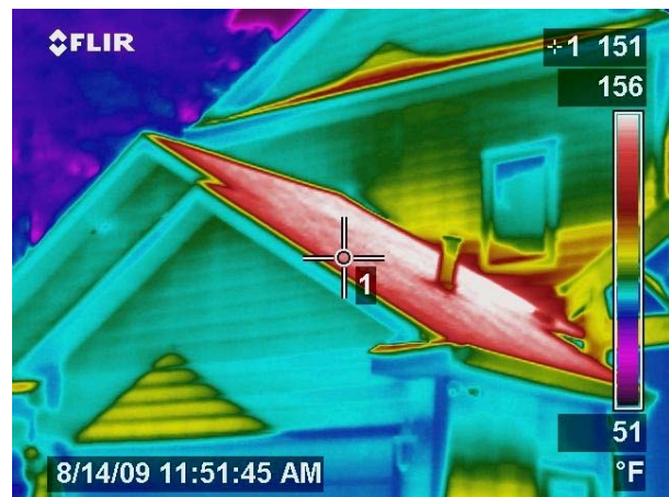
Figure 105 IR image of attic over garage. East-facing roof is about 151deg. F just before noon.
