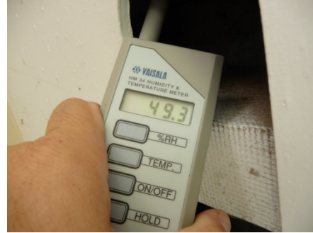
Figure 128 Measurement of RH (%) showing low humidity air discharging from the soffit vent on the south side of the house.
