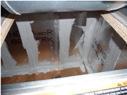
Figure 66 Inside of return plenum after repair.
