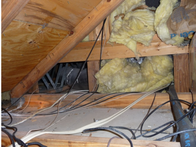
Figure 27 Garage attic open to interstitial floor space.
