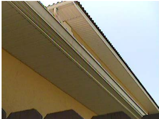
Figure 89 North vented soffit.
