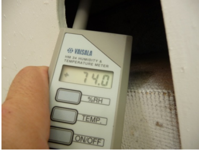
Figure 127 Evidence of cool, dry air emanating from the vented eaves on the south side of the house. (T)
