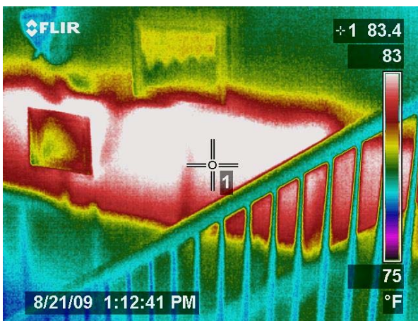
Figure 13850 Open floor cavity area in the east attic.
