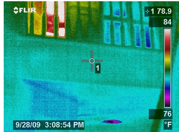
Figure 44 After repair, evidence of wind washing heat penetration into house interstitial cavities is now gone.
