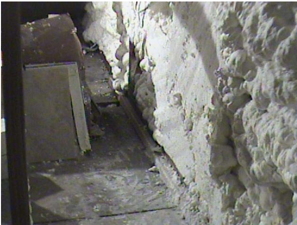
Figure 112 Floor post retrofit has been completely sealed and insulated.
