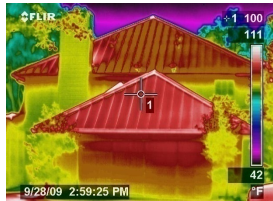
Figure 46 Roof in excess of 100°F. The bonus room is located in the center of the garage attic space.
