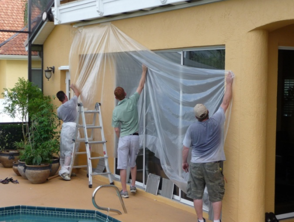
Figure 100 Preparation before foam installation to protect wall and glass from overspray.
