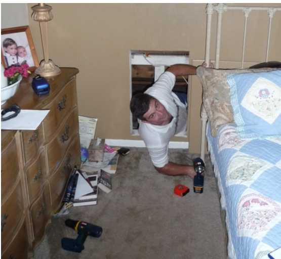
Figure 3 House H13. Visual inspection in the attic space is necessary to identify the presence and magnitude of wind washing.
