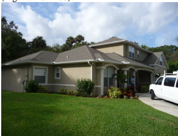
Figure 167 Front northeast view of home.
