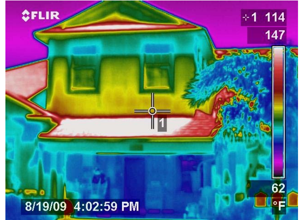
Figure 55 H7 Infrared image of west facing front taken August 19 about 4 PM.
