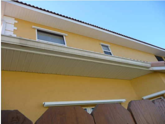
Figure 85 North attic is next to open floor space
