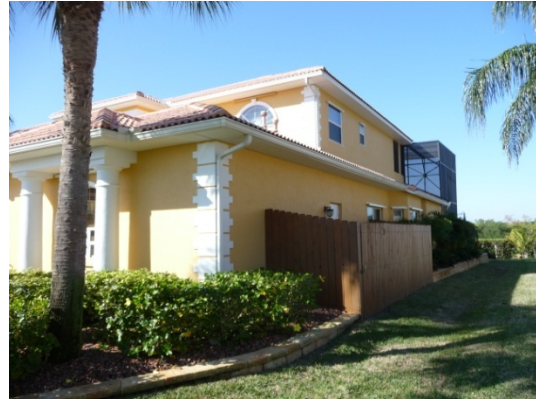
Figure 86 NE corner of house.
