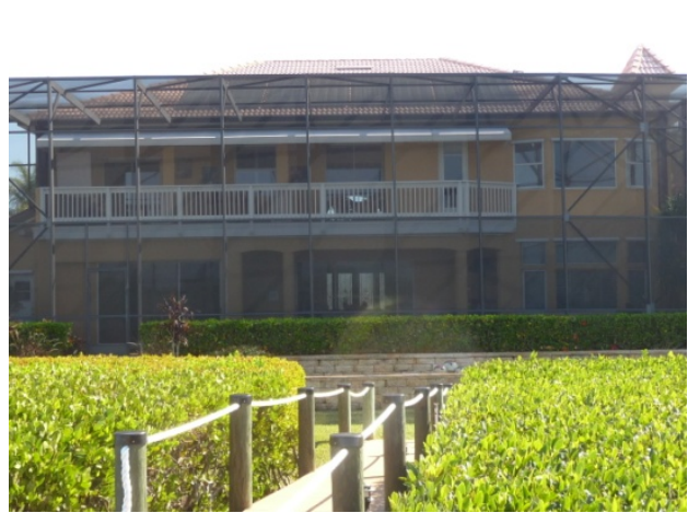
Figure 82 West back side of house
