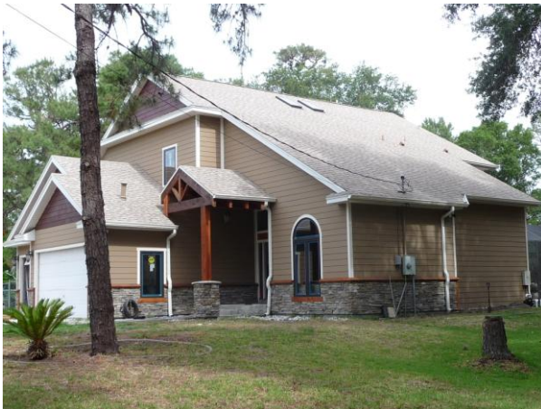
Figure E-11 Attic over garage faces south in house H16B.
