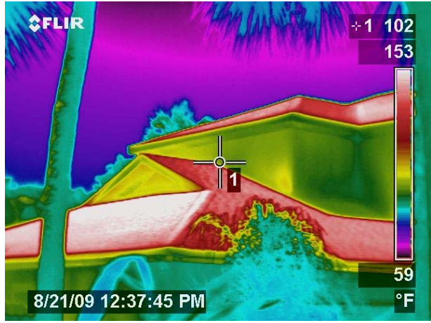
Figure 135 Infrared image of the house during midday after mostly sunny conditions all morning.
