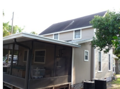
Figure 70 Back of residence.
