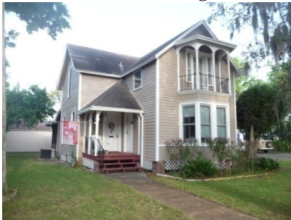
Figure 69 Front façade (front door facing East).
