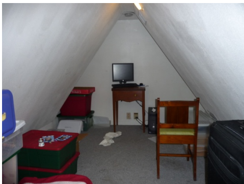
Figure 25 Bonus room with steep pitched wall/ceiling assembly
