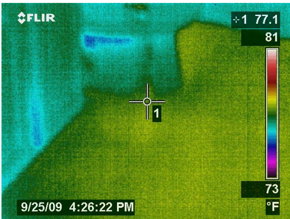
Figure 62 IR image of 2 nd story bathroom floor after repair. Floor surface is about 1.2°F cooler than pre-repair.
