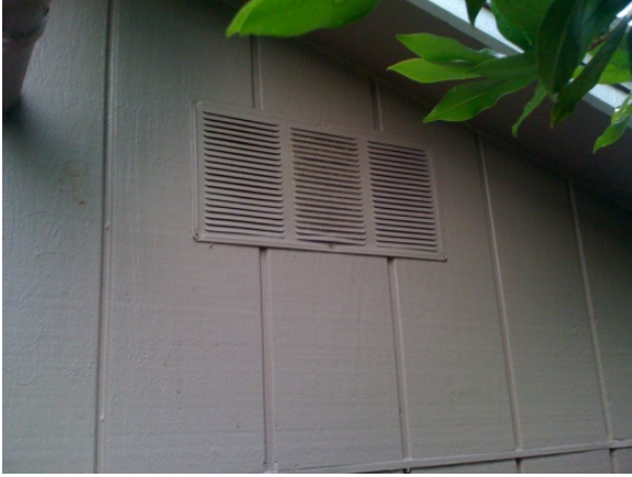
Figure 71 Gable vent view from outdoors.
