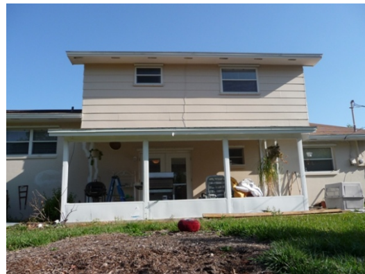
Figure 115 Back of home (facing south) with top story floor space cantilevered and vented over patio.
