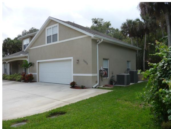
Figure 168 Northwest corner of home shows bonus room over garage.
