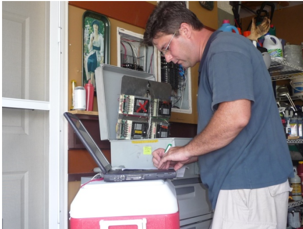
Figure 21 H8 Installing datalogger program and connecting sensor wires to datalogger.
