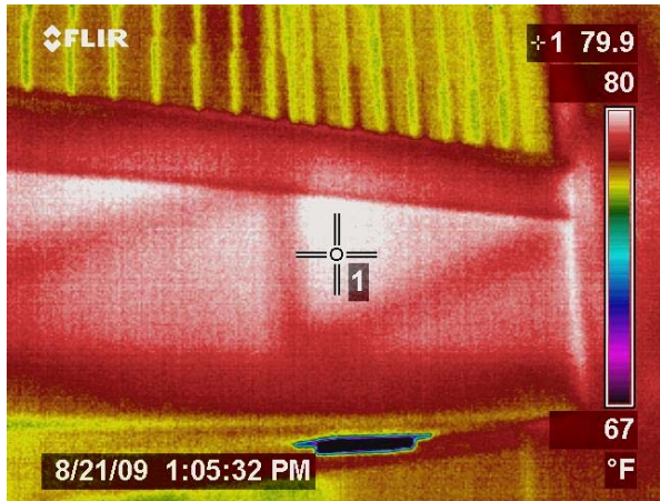
Figure 14052 Open floor cavity area in the east attic.
