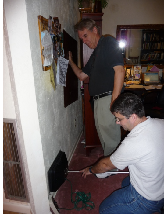
Figure 9 In House H5, a pressure pan measures return leakage in a wall cavity indicating substantial return leakage.
