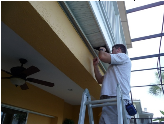
Figure 87 Rear (west) soffit access
