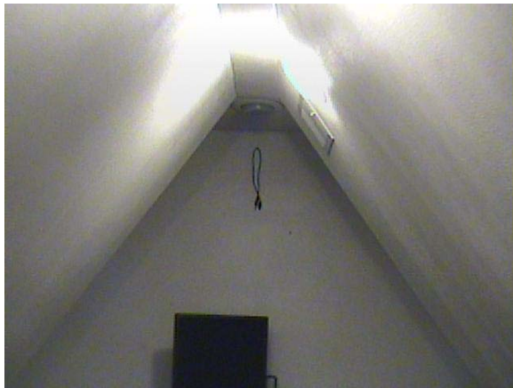
Figure 41 Ceiling and east wall of bonus room.
