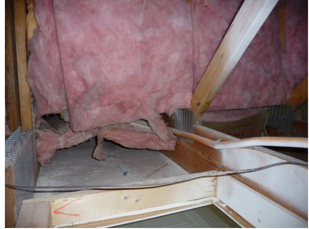
Figure 170 Open section of bonus room floor space near garage attic access.
