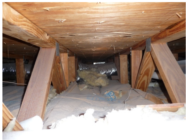
Figure 109 View inside floor space.
