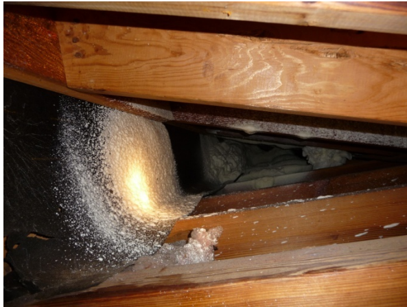
Figure 123 Beginning of north side sealing.
