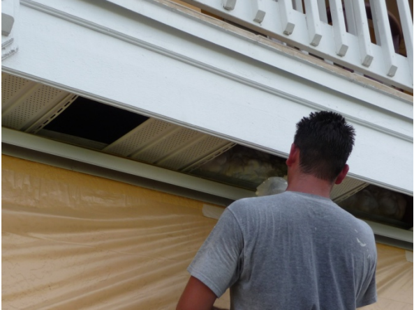
Figure 101 Foam application into west soffit area.
