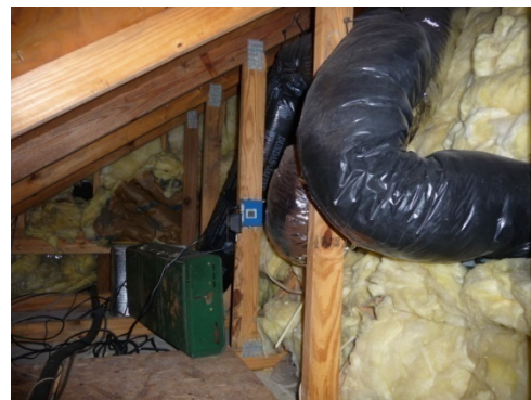
Figure 26 One side of bonus room wall as seen from attic space.
