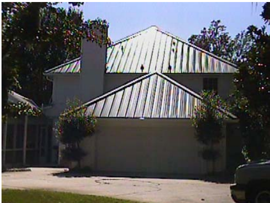
Figure 45 Garage with standing seam metal roof.
