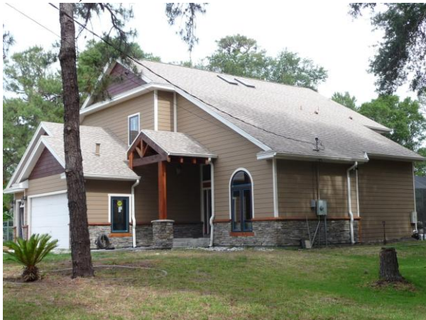
Figure 104 Attic over garage faces south.
