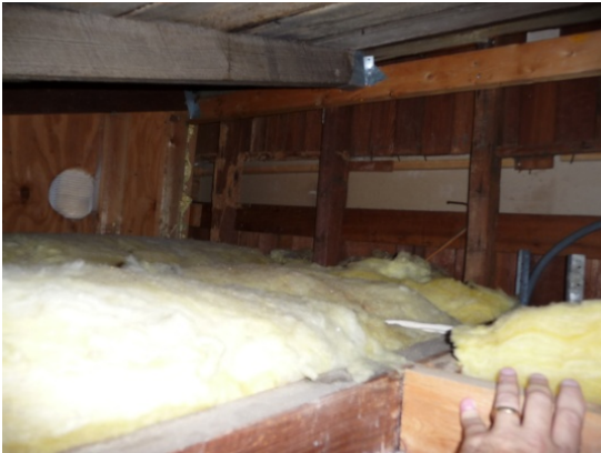
Figure 73 Photo of attic space with gable vent (left circle).
