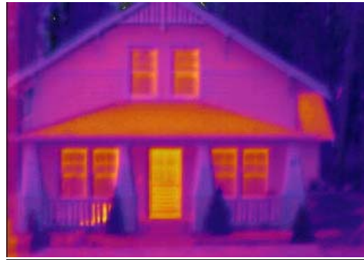
Figure 3- 31 Infrared Image of Brotherton 13th Ave Bungalows
