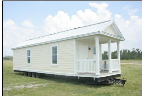
Figure 2- 5 FAS Emergency HUD Code Home for Mississippi
