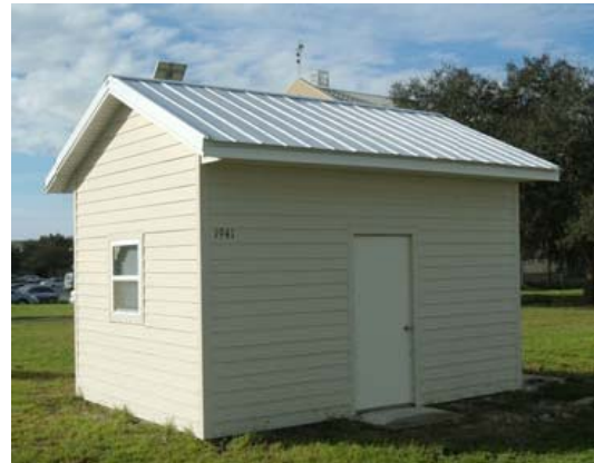
Figure 1- 24 NightCool Shed with White Metal Roof
