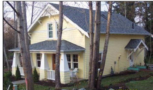
Figure I- 20. Brotherton 13th Ave Bungalows by Scott Homes, Olympia, WA.
