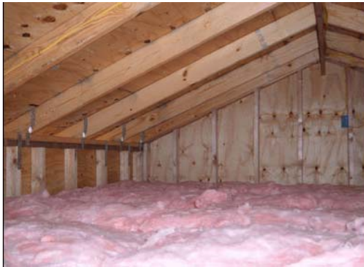
Figure 1- 234 Conventional Shed with Vented Attic and R-30 Fiberglass
