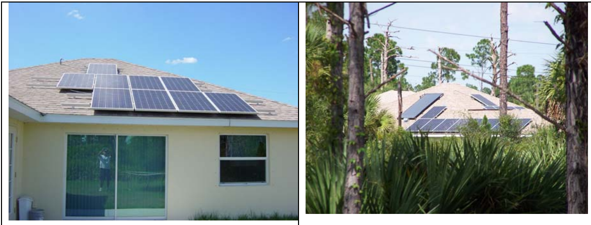
Figure I- 9. The Schroeders Homes NZEH in North Port, FL. The PV array is split on south and west roofs. Trees shade part of the array and the solar DHW collector in the afternoon
