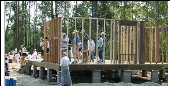
Figure I- 22. Raising Walls at a Habitat :”blitz build” in Slidell, Louisiana.
