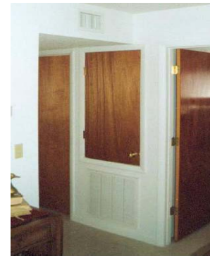
Figure 4- 7 An interior air handler, return plenum and supply duct chase
