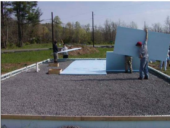
Figure 4- 21 Rigid insulation being installed on rock bed within ICF stem wall
