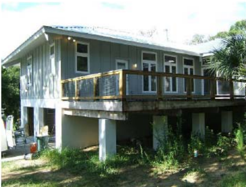
Figure 2- 11 Back view of Marquis Construction home in Dade City, FL
