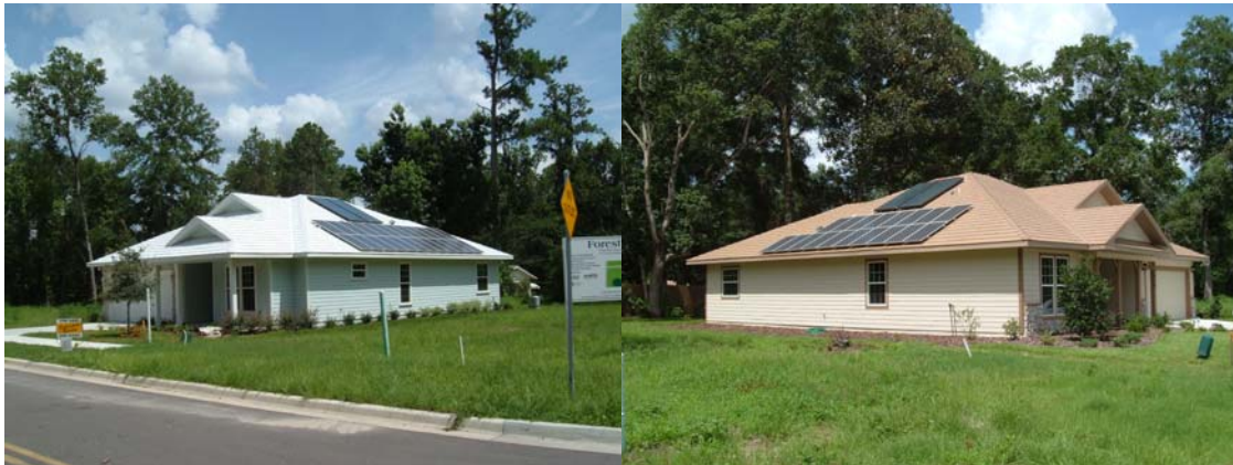
Figure 2- 18 Zero Energy and Near Zero energy Community Prototype Home, Gainesville, FL
