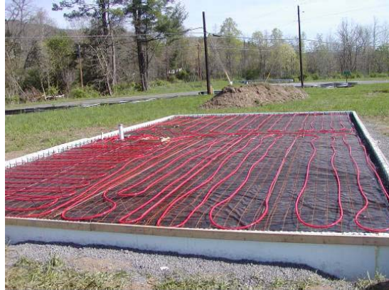
Figure 4- 22 Radiant floor system installed prior to slab pour
