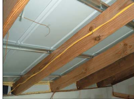
Figure 1- 25 Exposed Metal Roof in NightCool Attic
