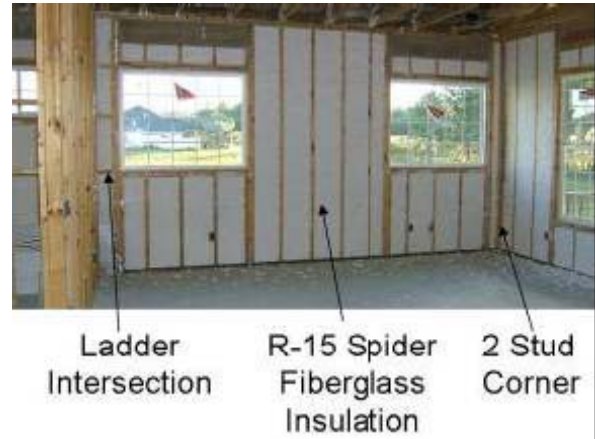
Figure 3- 18 Details reduce framing fraction and improve comfort.
