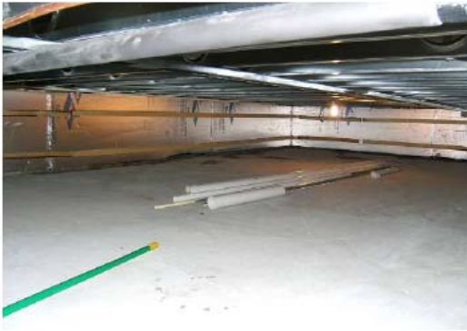
Figure 2- 9 Weather tight and insulated crawlspace
