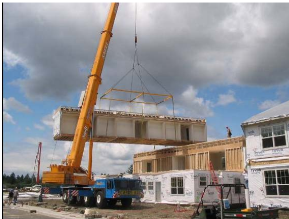
Figure 3- 28 Two Story Modular Housing Assembly, Ft. Lewis Army Base, WA
