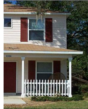
Figure 4- 8 Low-E windows are enhanced by 2ft overhangs, porches and site shading.
