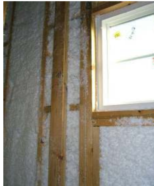
Figure 3- 19 Close up of ladder detail at the intersection of an interior wall. “Rungs” provide drywall nailing surface without compromising insulation.
