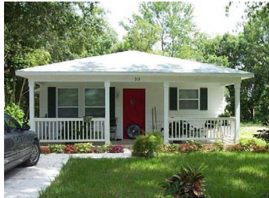
Figure I- 21. Lakeland, FL Habitat House conducting blower door testing.
