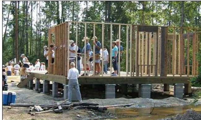
Figure 4- 16 Raising Walls at a Gulf Coast Habitat Build
