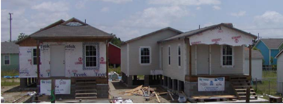
Figure 4- 20 New Orleans Area Habitat 30% Prototypes – both failed the TBIC.
