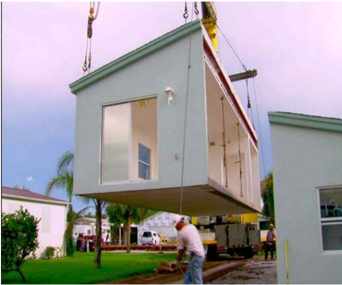
Figure 2- 16 Royal concrete concepts modular section
