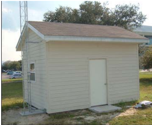
Figure 1- 22 Conventional Shed with Dark Shingle Roof
