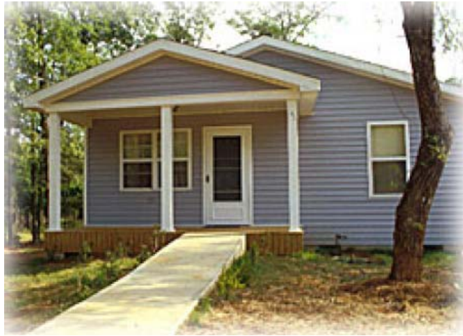
Figure 4- 1 Typical US Habitat for Humanity home; average costs $60,000
