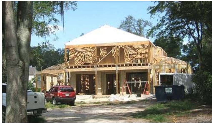
Figure 2- 15 Oyler Residence stem wall under construction.
