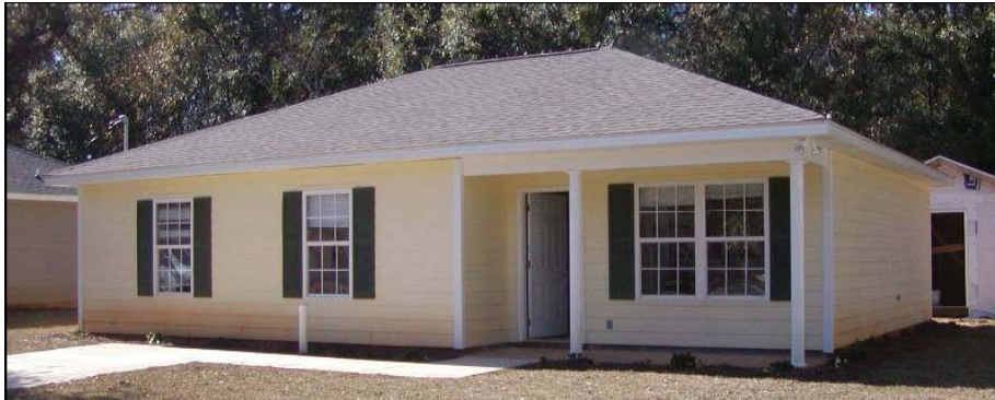
Figure 4- 3 Mobile County Habitat Home
