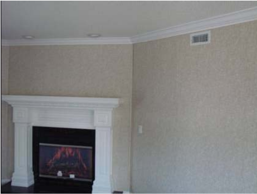
Figure 1- 1 High Side Discharge Vent Systems – Cavalier Homes
