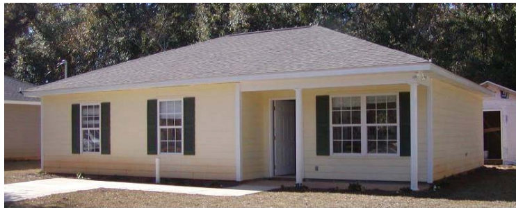
Figure 4- 19 Mobile County Habitat Home
