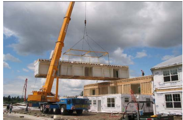
Figure 3- 4 Two Story Modular Housing Assembly, Ft. Lewis Army Base, WA
