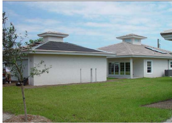
Figure 2- 25 Homes with solar hot water and BIPV on detached garage (not installed yet)
