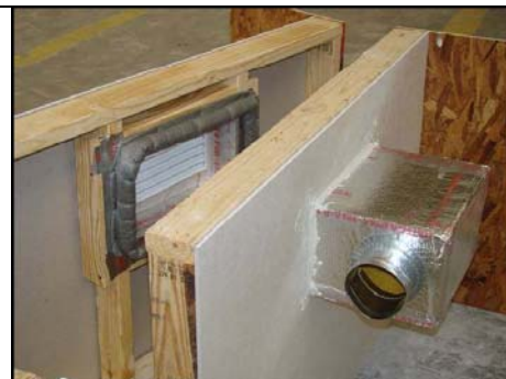
Figure 1- 5 Southern Energy Homes Interior Crossover Duct Mockup
