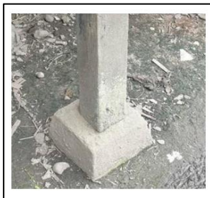
Figure 4 Mortar foundation
