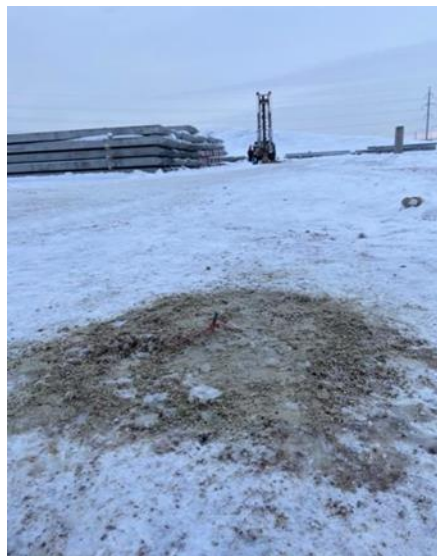
Figure 6. An antifreeze reagent on frozen ground
