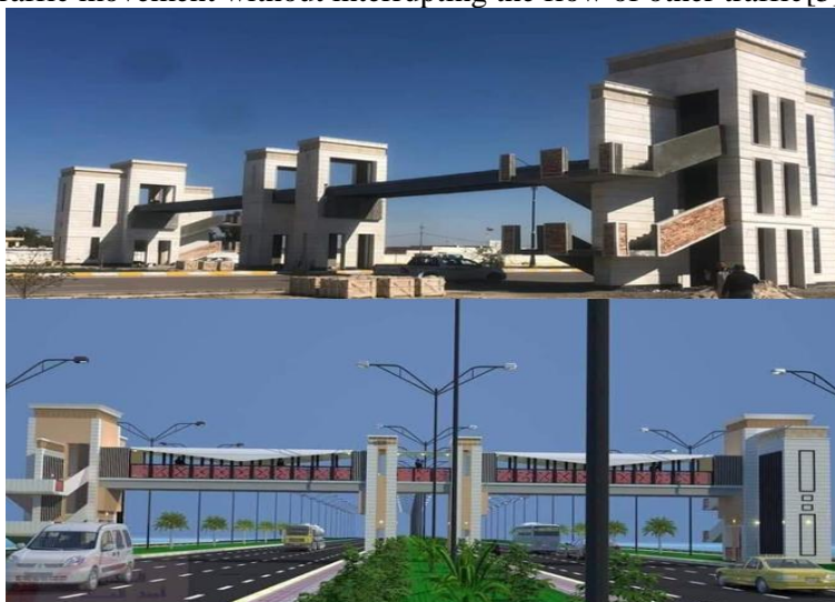
Figure 3. Structure of a pedestrian bridge in Anbar, Iraq
