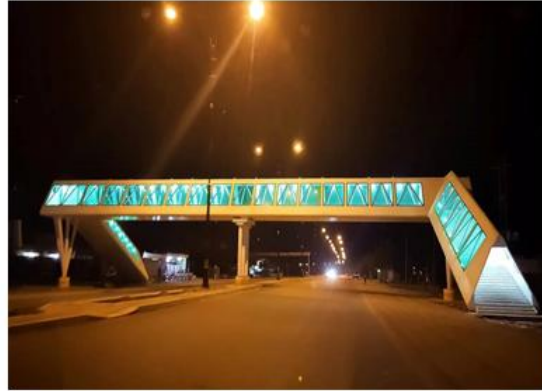
Figure 8. Streamline between the entrances and exits of the bridge with the surrounding space, as well as the aesthetic lighting at night (researchers)
