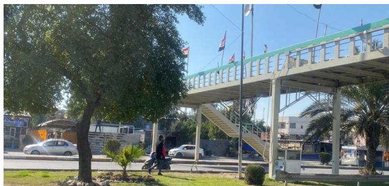
Figure 1. Visual aspects of the pedestrian bridge in Baghdad, Palestine Street
