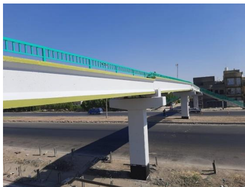
Figure 7. Locally manufactured iron quarries and the lack of color coordination with the environment
