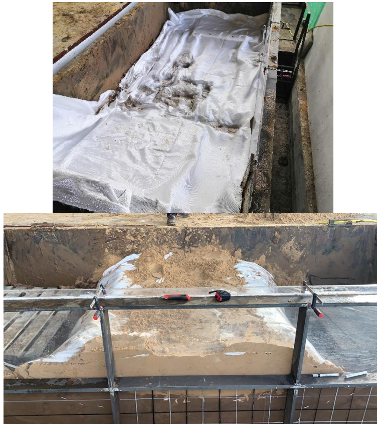
Figure 4. Formation of a reinforced soil holder at the base of the bridge on a "weak" base
