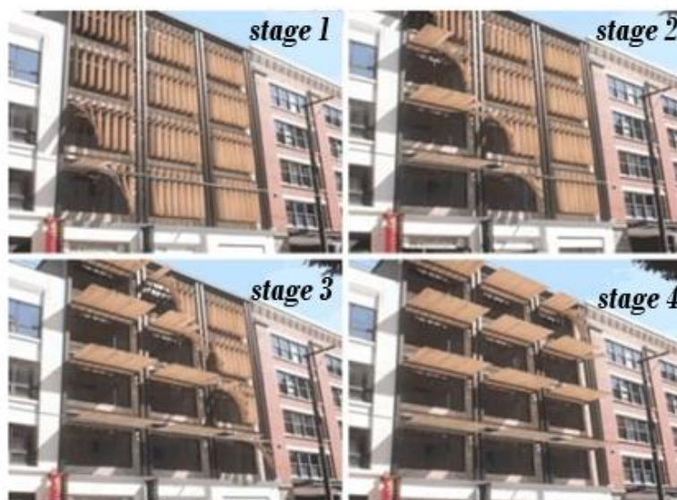
Figure 9. External curtains at the University of Oregon [25]
