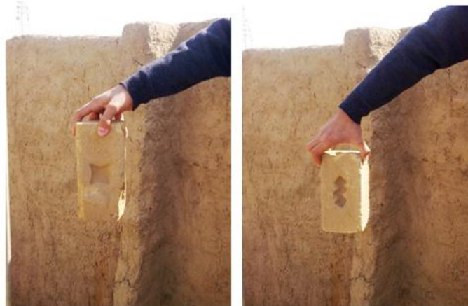
Figure 5. The shape of the bricks used in the traditional house (photographs by researchers)
