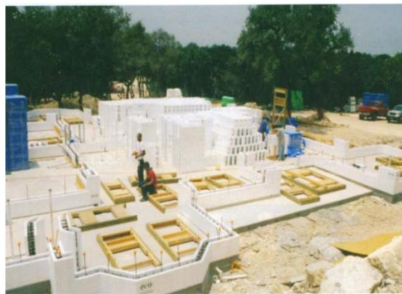
Figure 3. Construction of a building using DCG & BLOCK_ ECO technology [15]
