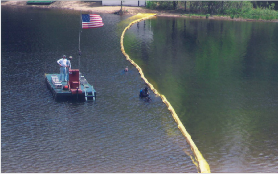
Figure 4. Installation of Herbicide Barrier Curtain
