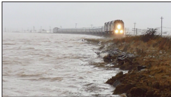
Figure 13. CN railway at Tantramar marshes on the New Brunswick–Nova Scotia border during high tide with storm surge of 60 cm, November 2015. Wave splash reached the rails. Photo by Mike Johnson, Cumberland Regional Emergency Management, reproduced with permission.
