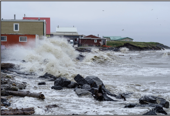
Figure 14. Waves breaking at Tuktoyaktuk, Northwest Territories, during a storm in August 2019. Coastal erosion at Tuktoyaktuk has forced relocation of houses such as these. Photo by Weronika Murray, courtesy of Natural Resources Canada.
