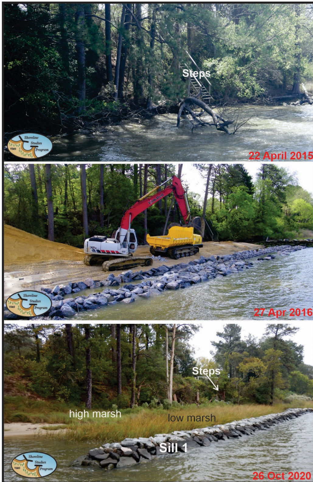
Figure 7-12. Pre-project shoreline showing an eroding bank with fallen trees (top); During construction of Sill 1 (middle); and Sill 1 about 4.5 years after construction showing a lush marsh (bottom). Photo credit: Shoreline Studies Program, VIMS.
