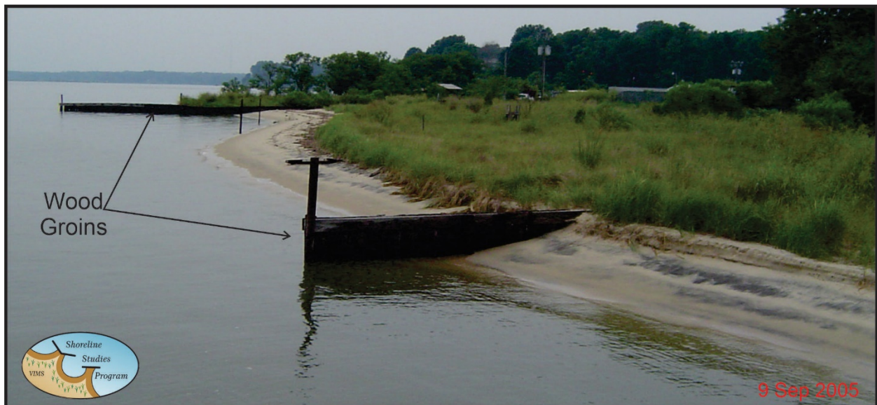
Figure 6-8. The VIMS West coast was a low eroding shoreline with wood groins for shore protection prior to installation of the breakwaters. Photo credit: Shoreline Studies Program, VIMS
