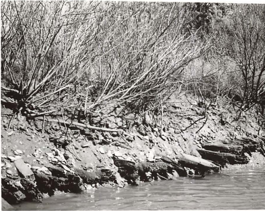
A. Corduroy road in Taskinas Creek marsh below farmhouse.
