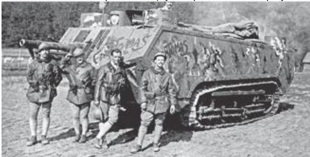
38. St. Chamond inadequate track. (By kind permission of Osprey Publishing).
