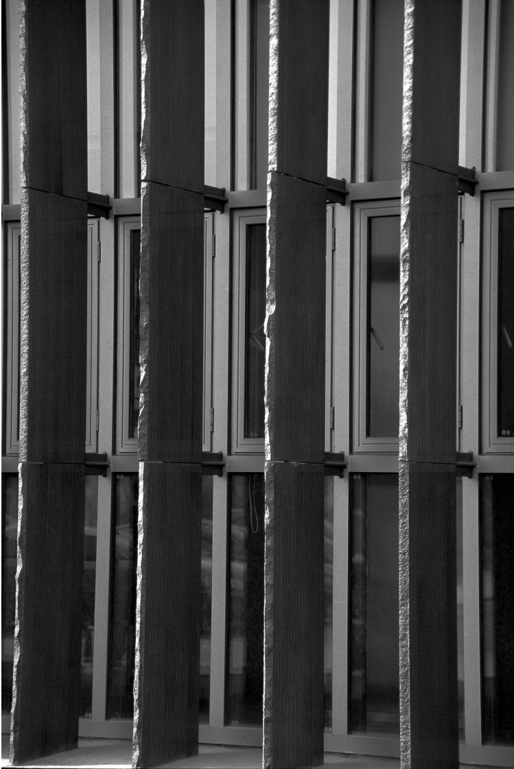
Figure 3.12 Liu Jiakun, Shanghai Qingpu District Exhibition Centre, Shanghai, 2006. Stone window shading
