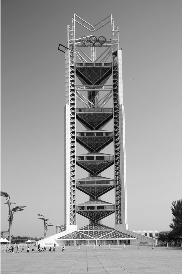
Figure 4.6 Cui Kai, Exquisite Tower, Beijing, 2008
