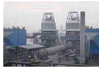
Fig. 17. Cement Rotary Kiln
