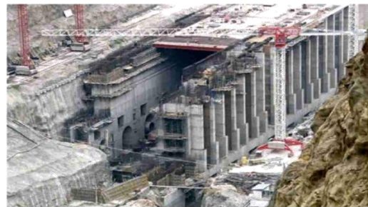
Fig. 24. Construction of thermal plant using Low heat cement
