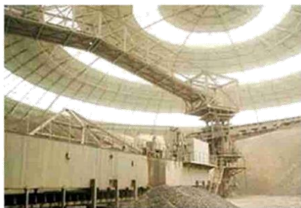
Fig. 10. Stacker and Reclaimer
