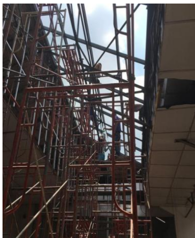
Gambar 6. Proses Renovasi Skylight Sumber: M Bloc Space, 2020.
