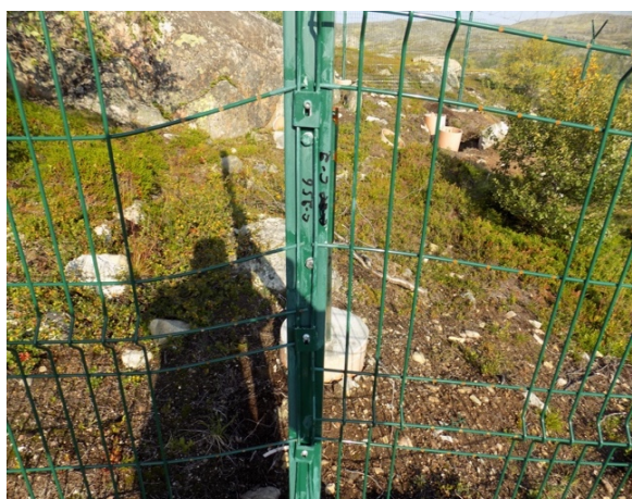
Fig. 3. Destruction of the panel near to the support.
