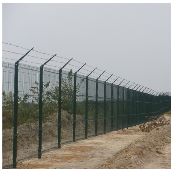
Fig. 1. View of an undamaged grating fence.
