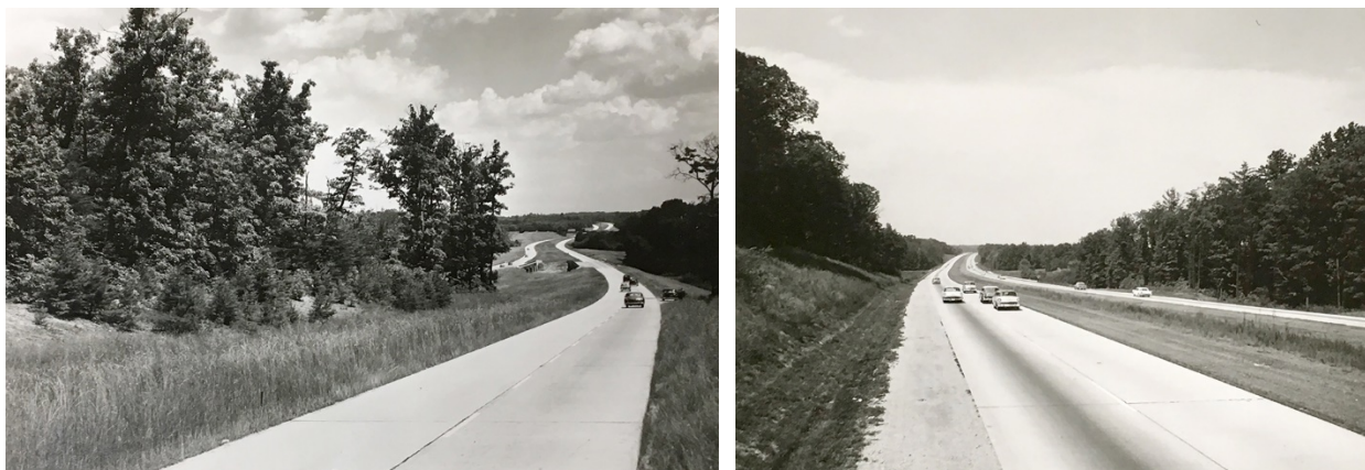
Fig. 2: Historic photos with parkway character (left) and highway character (right)
