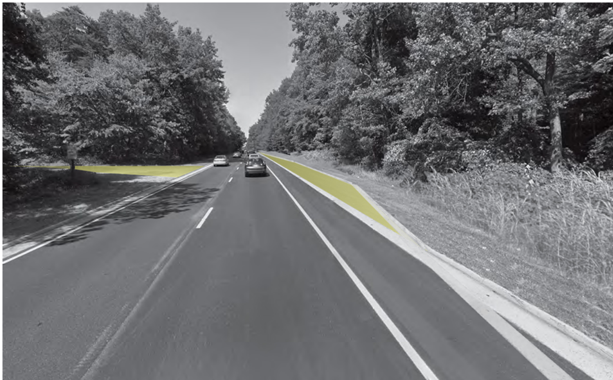
Fig. 7: Emergency pull-off and crossover with grass pavers to minimize visual impact.
