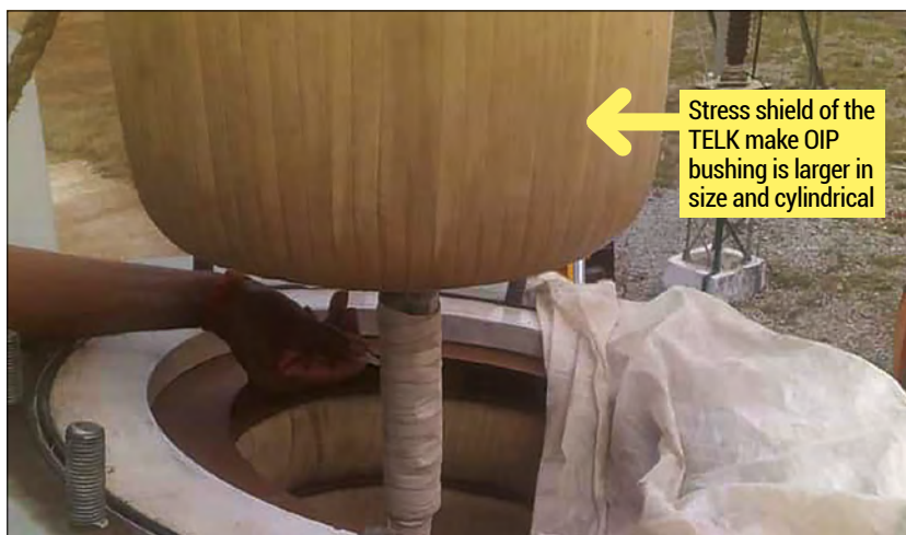
Figure 8. A 420 kV OIP TELK's design bushing being inserted through the turret with a stress shield
