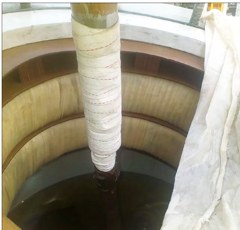
Figure 9. Cotton tape wrapped over the half-lap joints of 1 V phase winding lead and the draw-rod type bushing, tightened
