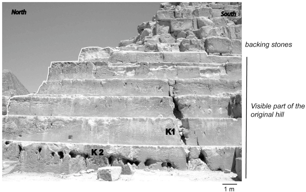
Figure 9. Khephren Pyramid. View of the northern part of the W face. The visible part of the original hill (delimited by the white line) shows horizontal steps without horizontal or vertical block breaks. K1: karst natural fracture, K2: discontinuities showing advanced dissolution processes along the strata surface.
