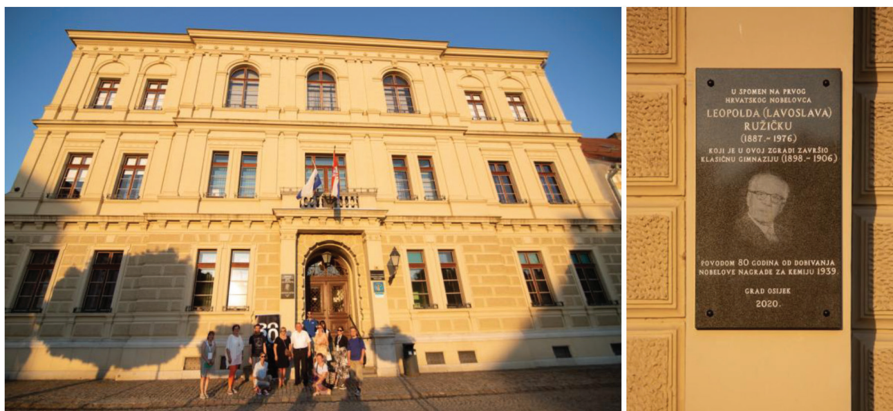
Fig. 2 – The building of Classical Grammar School in Osijek, today's Economic Administrative High School with the plaque dedicated to Ružička
