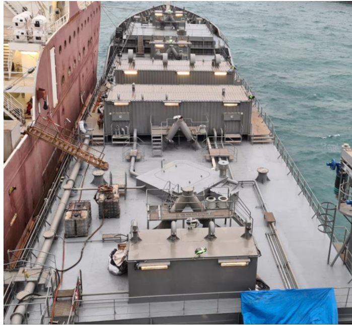
Figure 11 Ship no.2 new cargo (cement) compression and blowers' units placed in the 40 feet specially designed containers placed on the existing hatch covers that are welded to the hatch coamings
