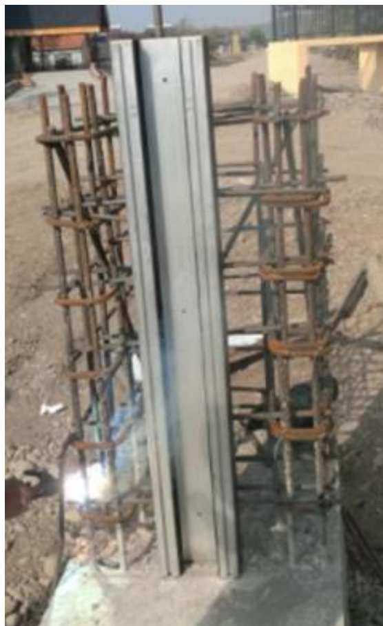
Figure 14. End post welded to the reinforcement.
