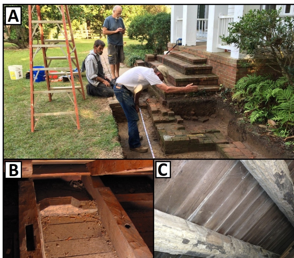
Figure 1. Walker House (A) pre-existing brick foundation, (B) hand-finished attic timbers, and (C) crawl-space oak joists. Photos by R. Doherty.
