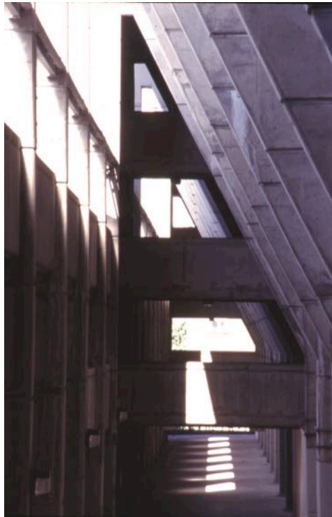
Figure 11.3 View through apex of concrete A-frame structure supporting housing block, with access level to atrium below
