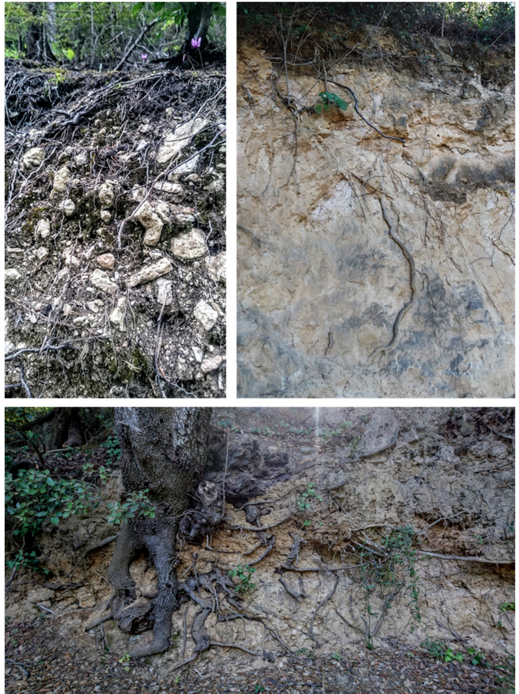
Figure 2. Interactions of small and large roots with soil particles and rocks that generate the root reinforcement effect.
