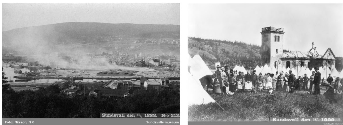
Figure 5.2. To the left; View over Sundsvall two days after the fire in June 1888. To the right; Tent camp for the homeless people after the fire of 1888. The burnt-down church Lovisa Ulrika was captured in the background. Digital Museum, 2021.
