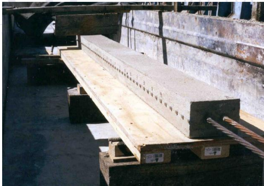
Figure 2.2: Concrete with metal points on the surface
