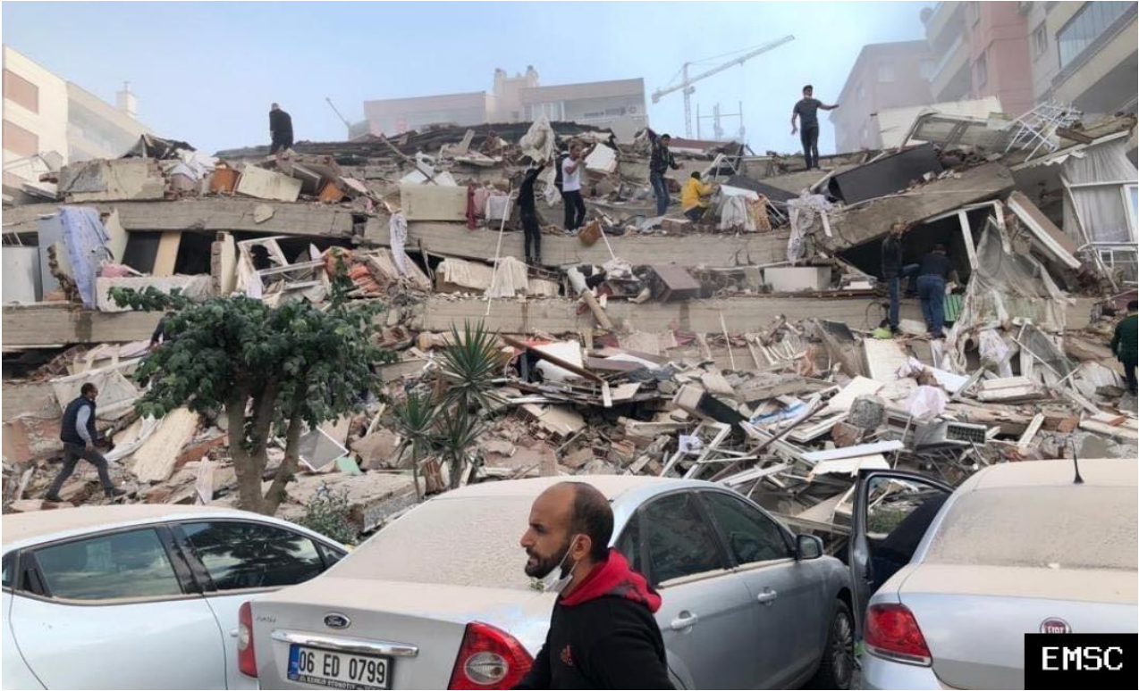
Collapsed building after the Aegean earthquake.
