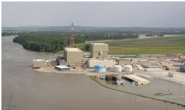
Figure 9. Missouri River flooding in June of 2011 reached the Omaha Public Power District’s Fort Calhoun Station, a nuclear power plant north of Omaha. From “Northern Great Plains” by Conant et al., 2018, Impacts, Risks, and Adaptation in the United States: Fourth National Climate Assessment, Volume II , p. 963. Photo credit: Harry Weddington, U.S. Army Corps of Engineers.
