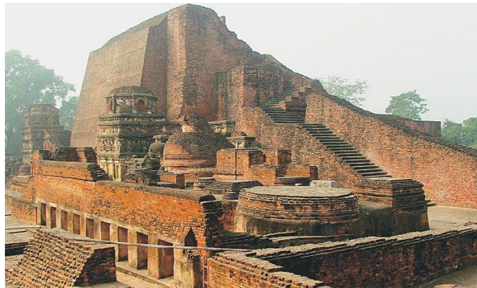
(Figure – 1. Great Monument. The stupa base in the foreground is imagined by some to be the location of Nalanda Library)
