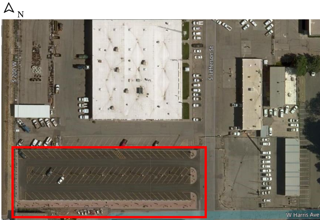
Figure 4: BR system at Salt Lake City Public Utilities, Salt Lake City, Utah
