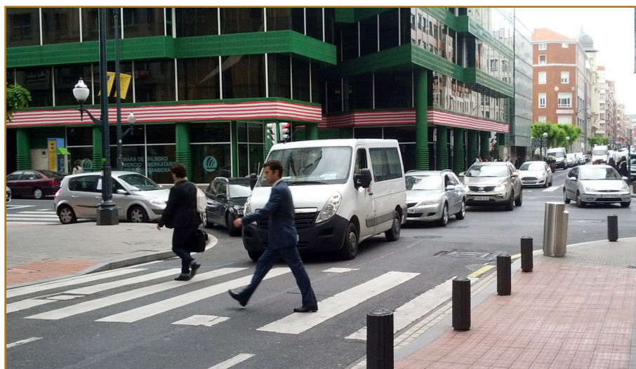
Unsignalized leg of partially signalized intersection.
