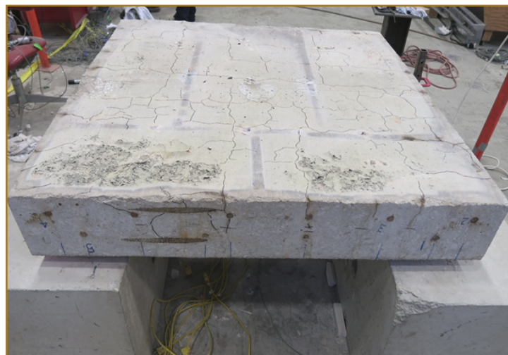
Deck specimen after heating.
