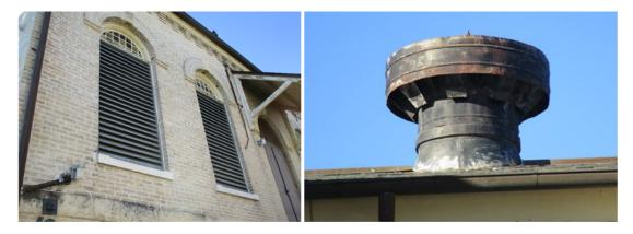
Figure 1: Building 615's historical attic vent and window to be restored. (Credit: Courtesy of Freese and Nichols)
