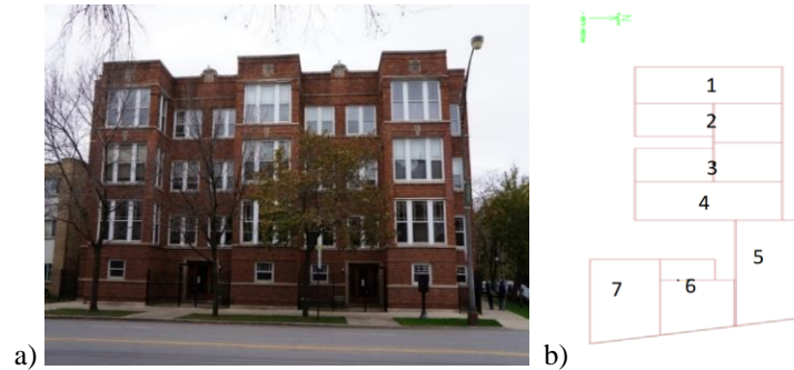
Figure 1: a) Real building East View, b) Building Floors plot including thermal zones positions
