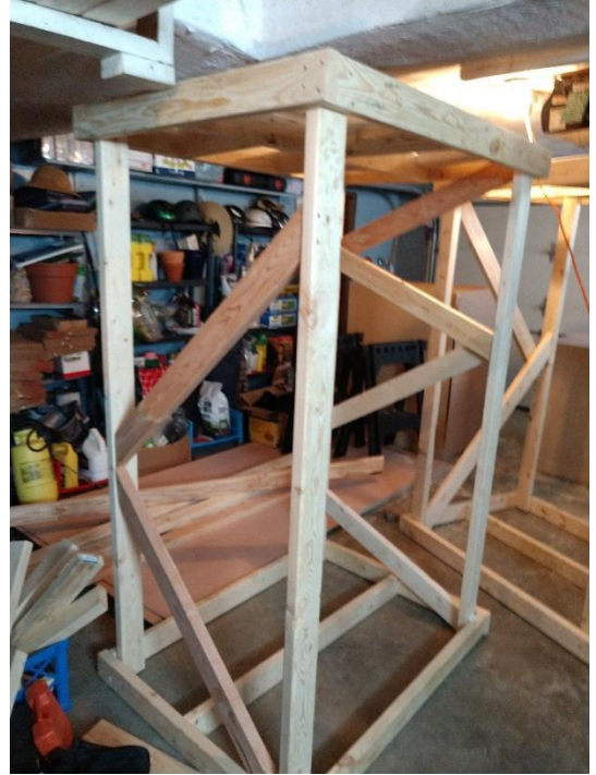
Figure 7 The bottom parts of the towers. These are each six feet tall and can support at least 250 lbs.
