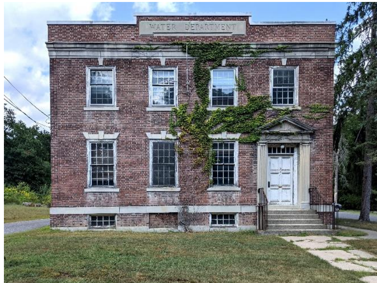
Figure 5: South Façade of Water Department Building
