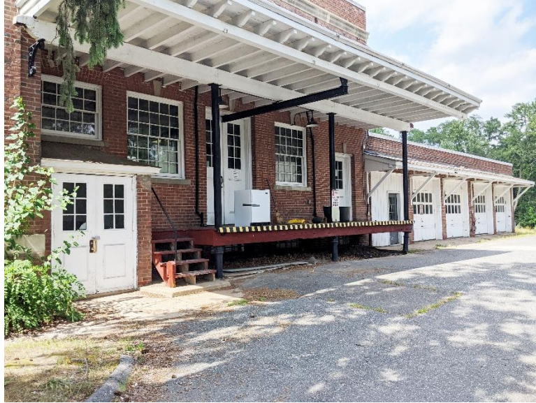
Figure 6: East Façade of Water Department Building
