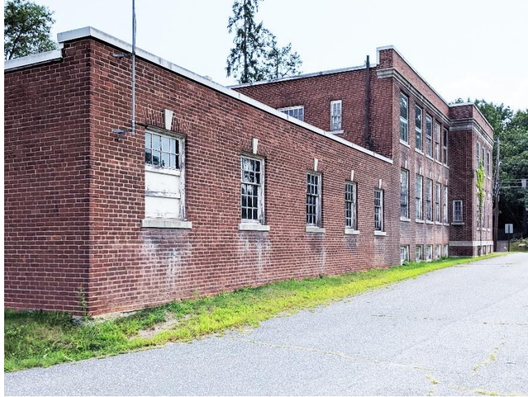
Figure 7: West Façade of Water Department Building
