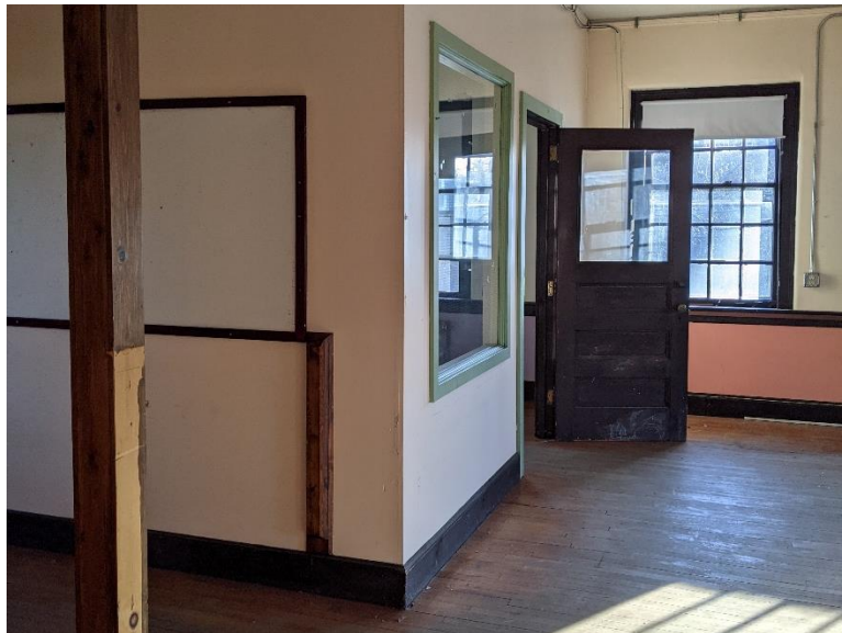
Figure 8: Front Section Interior
