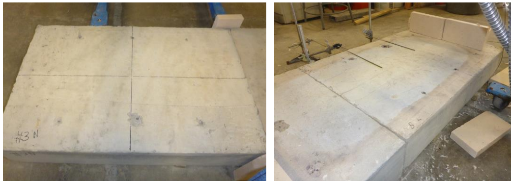
Figure 7.21: Slab before heating (left), whitening after heating to surface temperatures up to 930°C (right)
