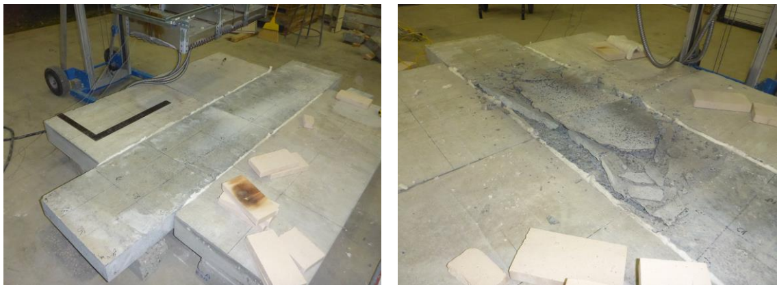
Figure 7.38: Spalling of 600°C beam specimen prior to heating (left), post heating (right)
