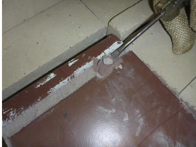
Figure 7.28: Removal of grout with a screwdriver after heating
