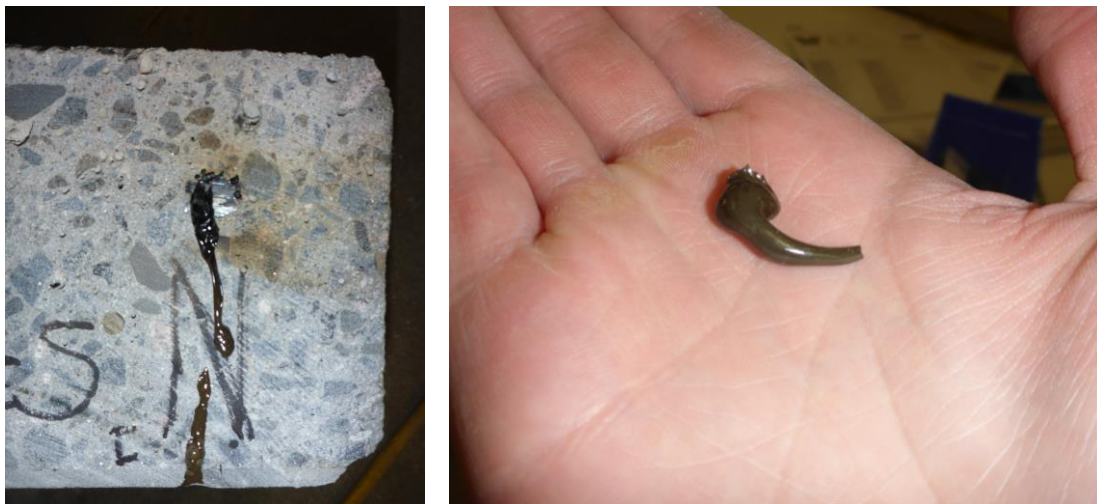
Figure 7.29: Melting of epoxy reinforcement coating
