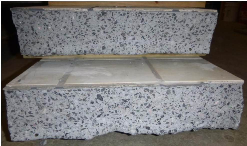
Figure 7.46: Ruptured surface of 300°C heated specimen
