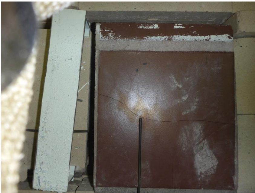
Figure 7.27: Closeup of tile and aluminum wireway after heating
