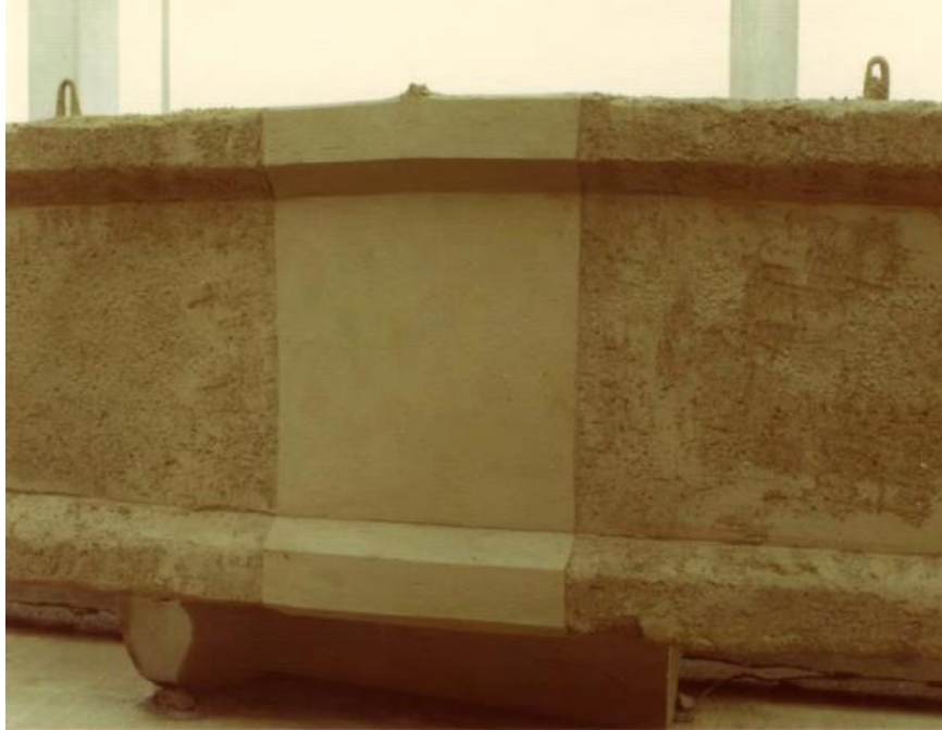
Figure 5.12: Midspan of the girder after repair (Reproduced from fib Bulletin 46, page 130 - “central part of the girder after shotcreting” by Taerwe et al. 2006, with permission from the International Federation for Structural Concrete (fib) [8])
