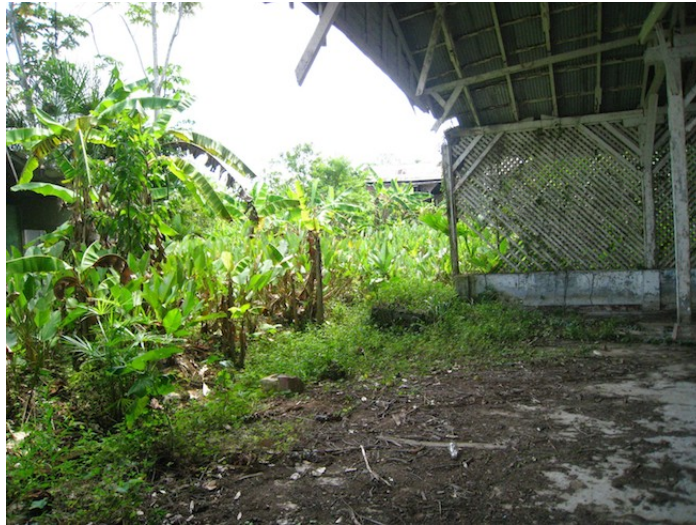
Figure 11. Overgrown sawmill infrastructure at former Astoria site Photograph by the author
