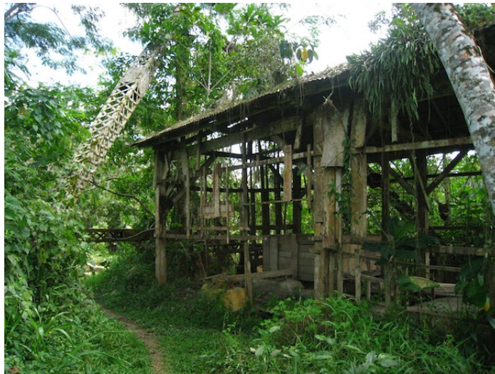
Figure 12. Rusted metal crane and overgrown sawmill infrastructure at former Astoria site Photograph by the author
